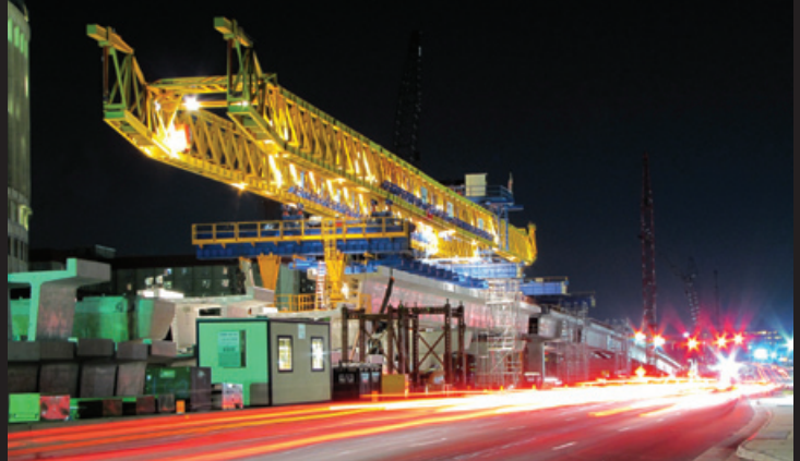
M.C. Dean (No. 14) is furnishing, installing, testing and commissioning the mechanical, electrical and plumbing systems on the Dulles Corridor Metrorail Project in Va., one of the biggest U.S. transportation projects.
